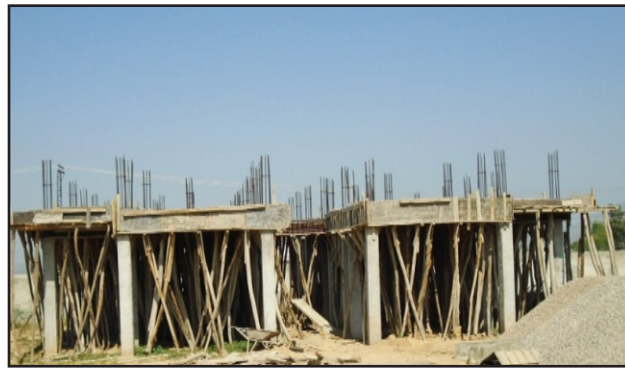
Photograph showing the progress of construction work on Faculty & Staff Residencies
