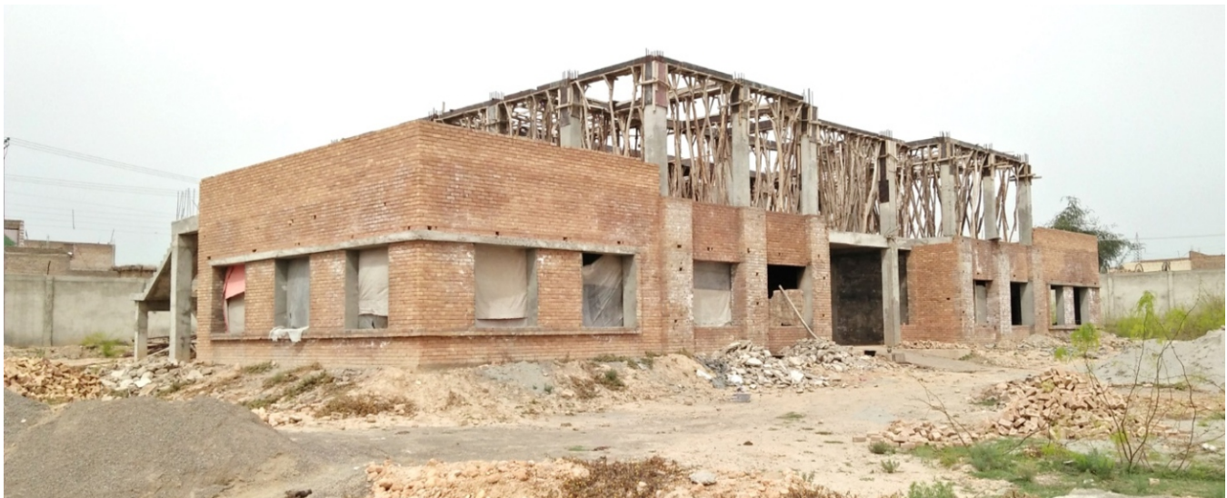
Photograph showing the progress of construction work on Central Library
