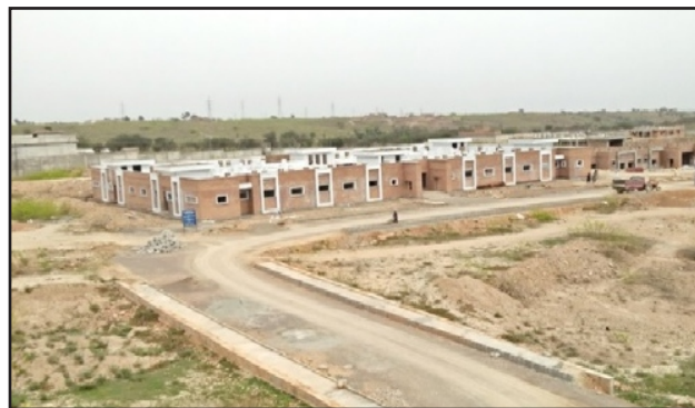
Photograph showing the progress of construction work on External Developments
