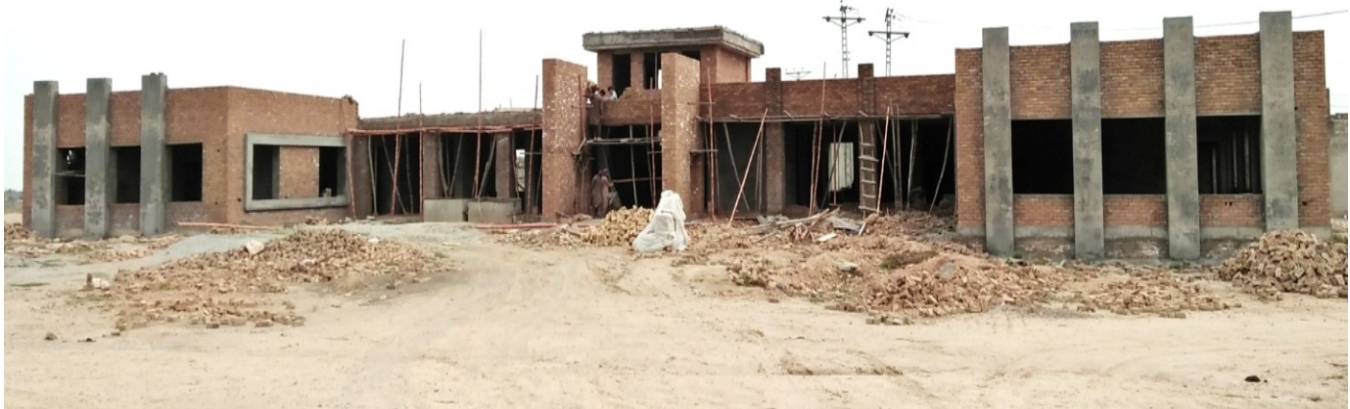
Photograph showing the progress of construction work on Common Facilities
