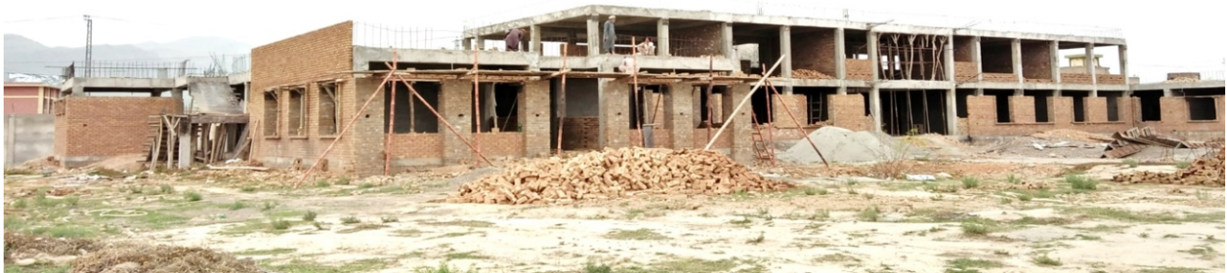
Photograph showing the progress of construction work on Admin Block
