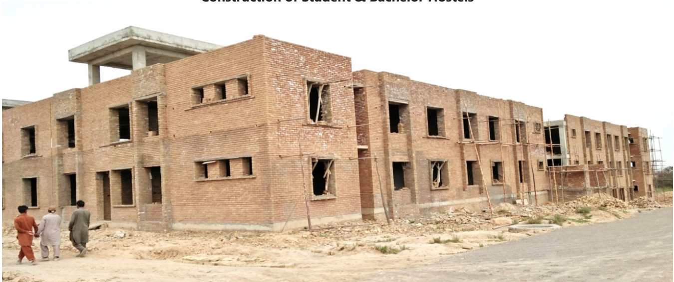
Photograph showing the progress of construction work on Boys Hostels
