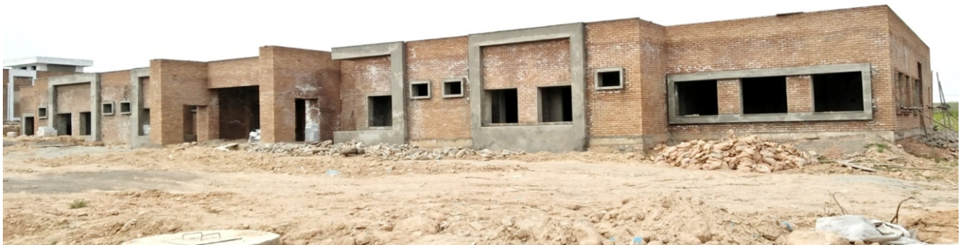
Photograph showing the progress of construction work on Faculty Hostels
